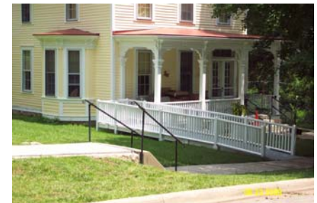
Modifications to structures for handicap accessibility shall respect the historic structure’s integrity
